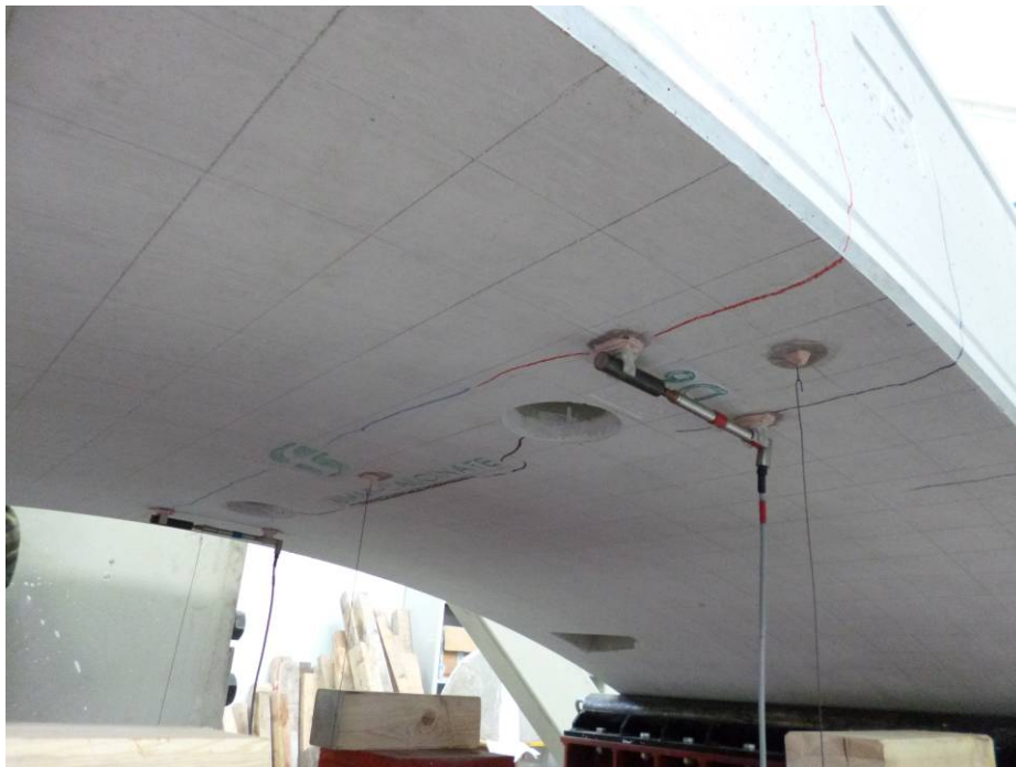
Figure 43. Segment D6: load level of 164 kN, intrados surface
