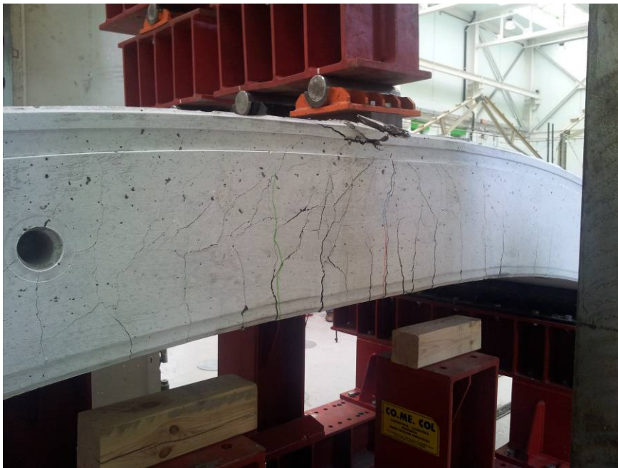
Figure 35. Segment D5: failure stage: left lateral surface.
