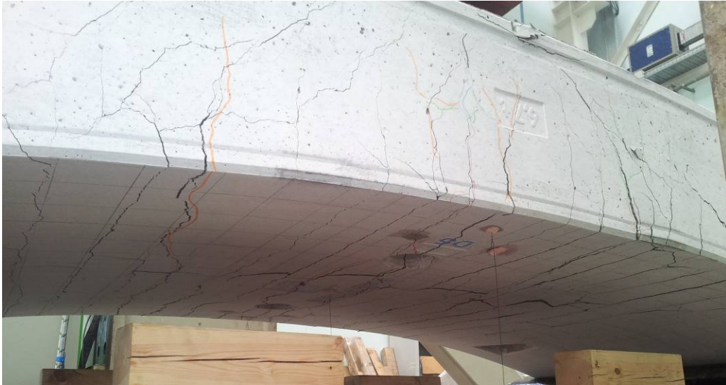
Figure 36. Segment D5: failure stage: intrados surface.
