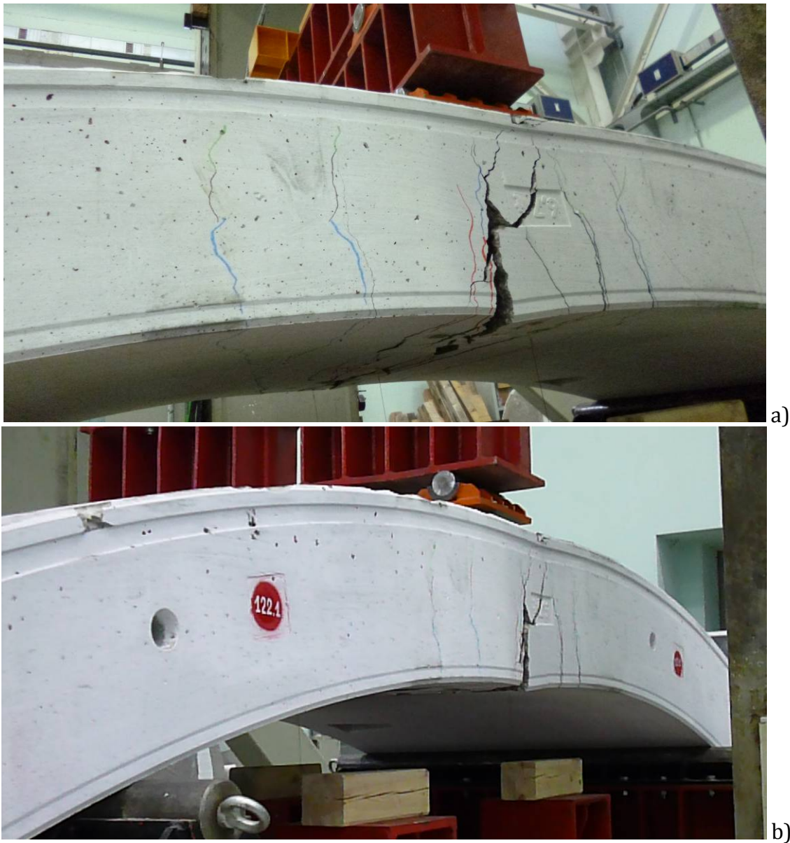
Figure 20. Segment D4: failure stage a) left lateral surface, b) right lateral surface.
