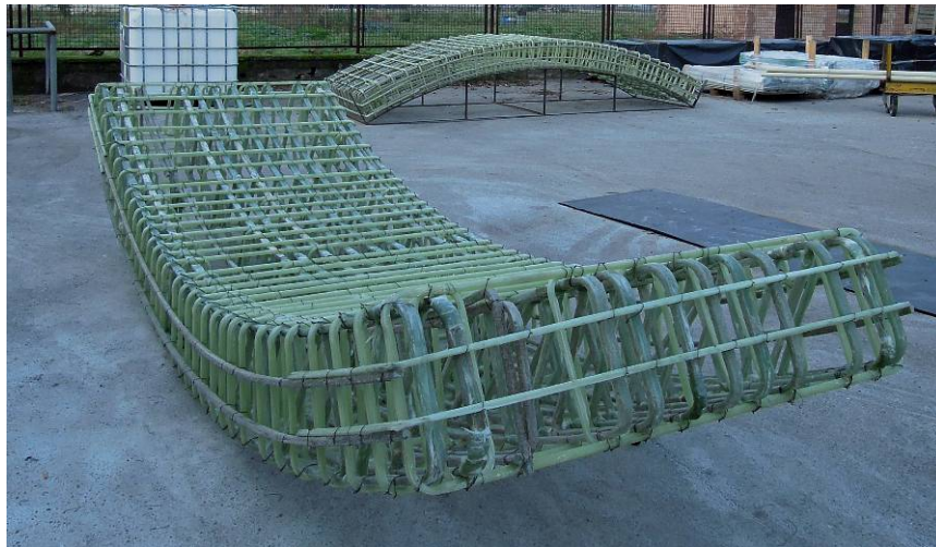
Figure 2. Segment D4: traditional steel cage
