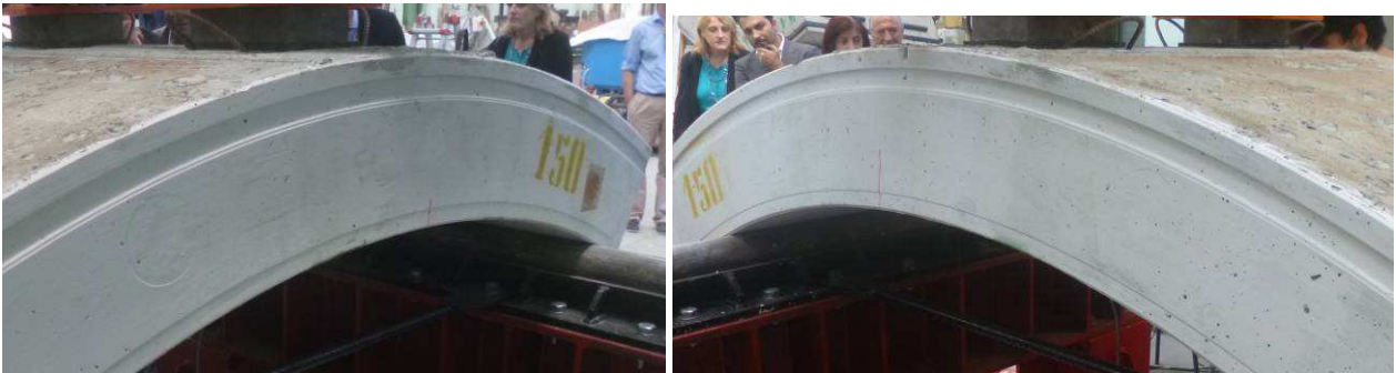
Figure 8. First crack, lateral surfaces
