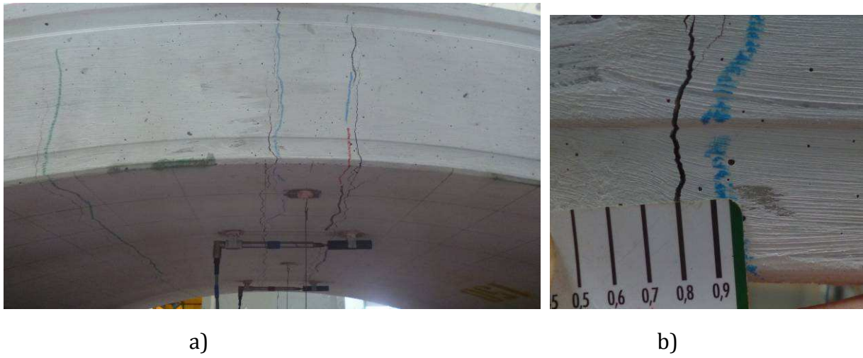
Figure 12. Load level 185 kN. Crack pattern; a) intrados, b) maximum crack width
